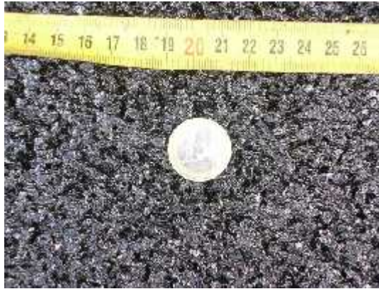
Figure 6. Crumb rubber modified asphalt concrete
